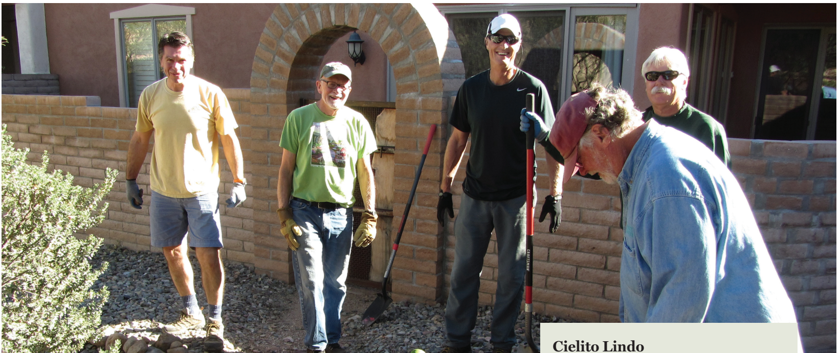
PHOTO: 2016 Repairing Storm Retention Ditch (courtesy Leo Francis)
