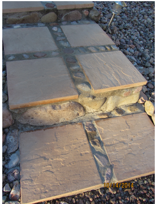
Example 3: Rock risers, Flagstone treads
