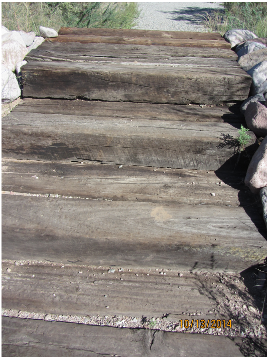
Example 2: Railroad tie risers and treads
