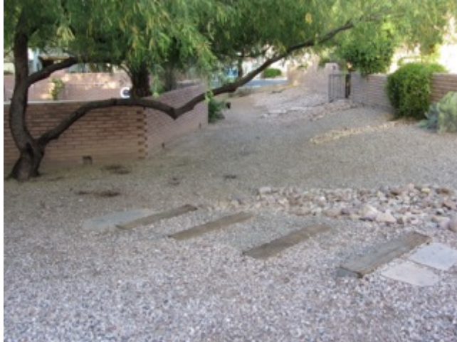
Example 1: Railroad tie risers with gravel treads
